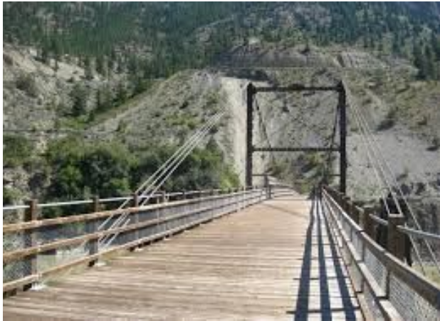
Old suspension bridge
